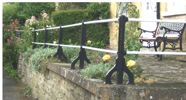
Cast iron railings along The Terrace
